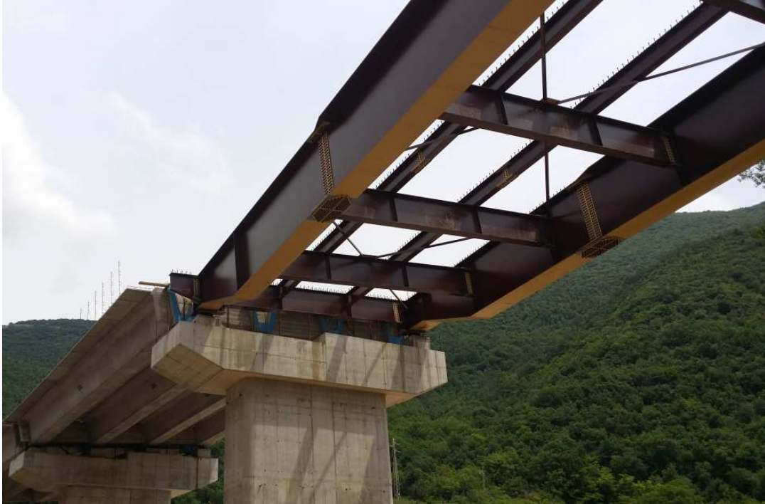
Figure 4.3: Girders installation. Visit to the ongoing works in the road between Perugia and Ancona, Italy.
